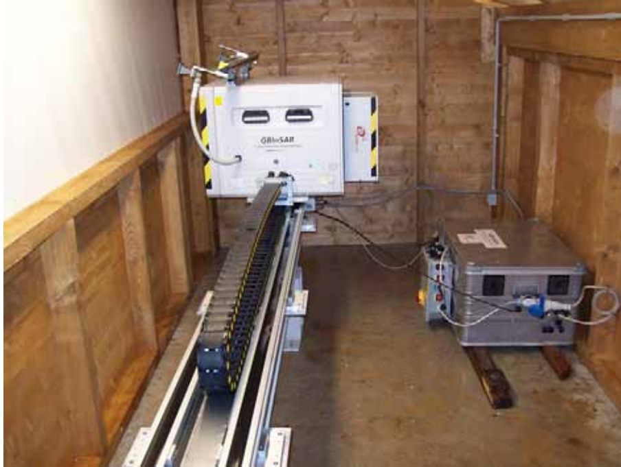
Figure 3.6: GBinSAR installed in a shelter on the Shara del Fuoco (Stromboli Volcano, March 2007).
