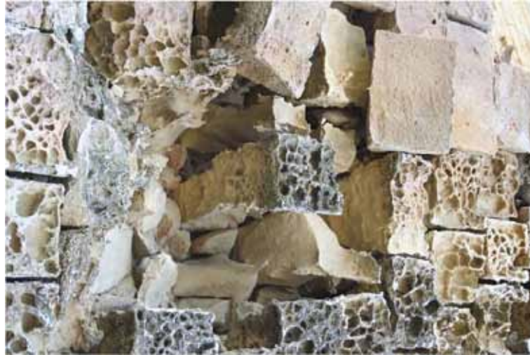
Figure 5.23: Detail showing the conditions of underwalling masonry structures (May, 2010).
