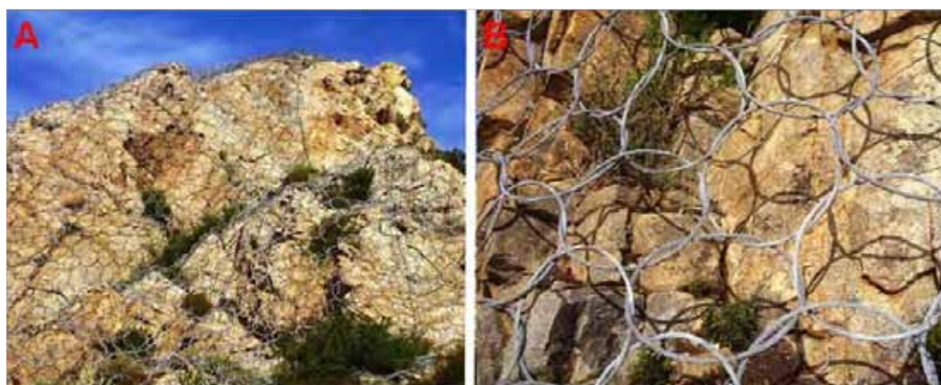
Figure 7.14: Boulder net with circular mesh installed in the period '99-'01 (April, 2010).
