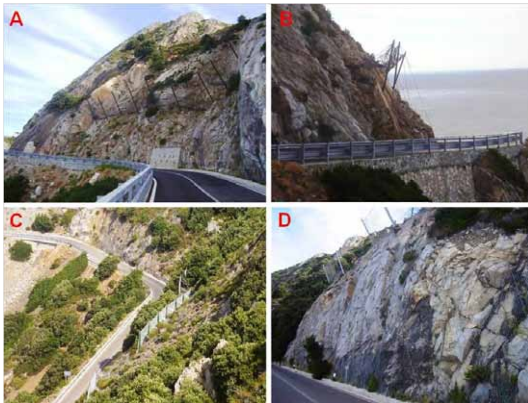
Figure 7.8: Section of provincial road N° 25 within the study area (March, 2010).
