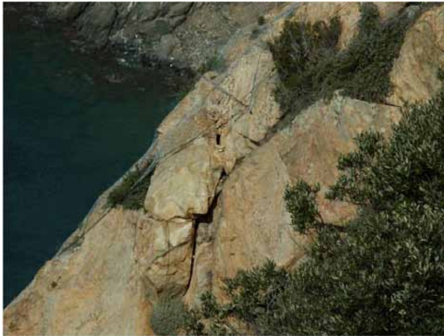
Figure 7.18: Unstable porphyry block located within the lower part of the rock mass 1 (May, 2010).
