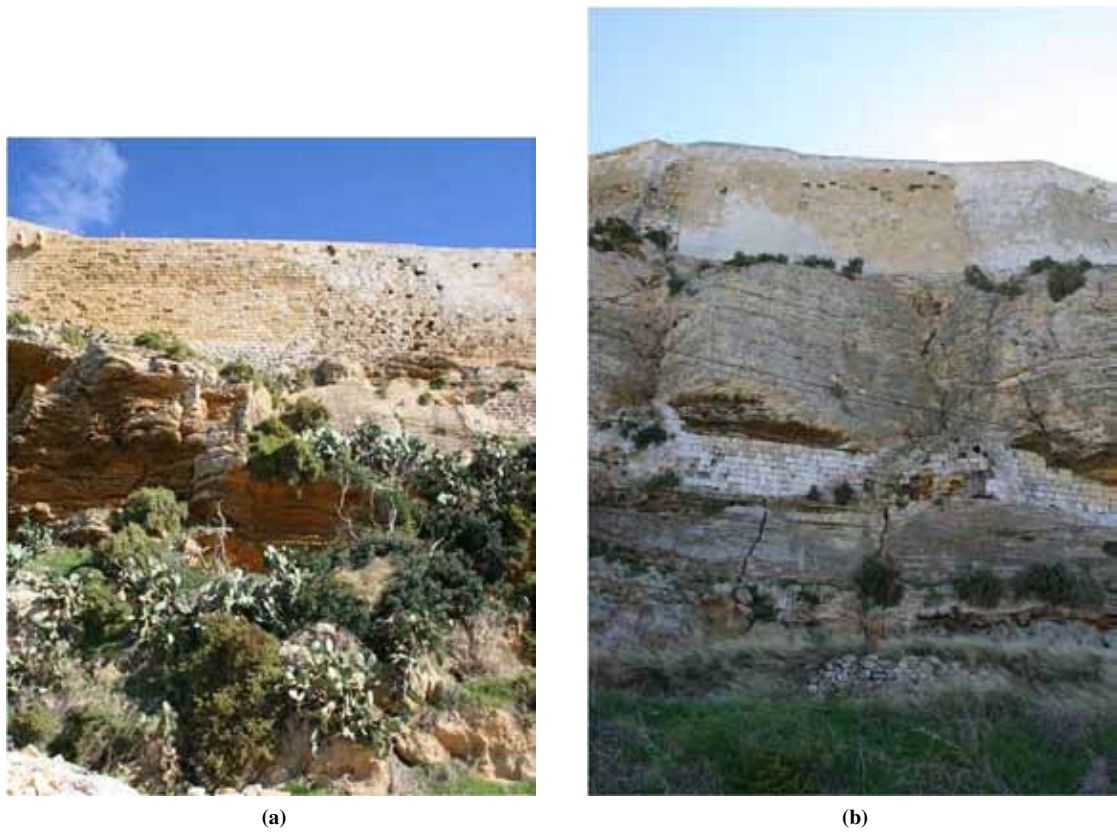
Figure 5.21: Gozo aut crops. a) Ledges and niches on the cliff due to differential erosion. b) High persistence joints within the rock mass (April 2009).
