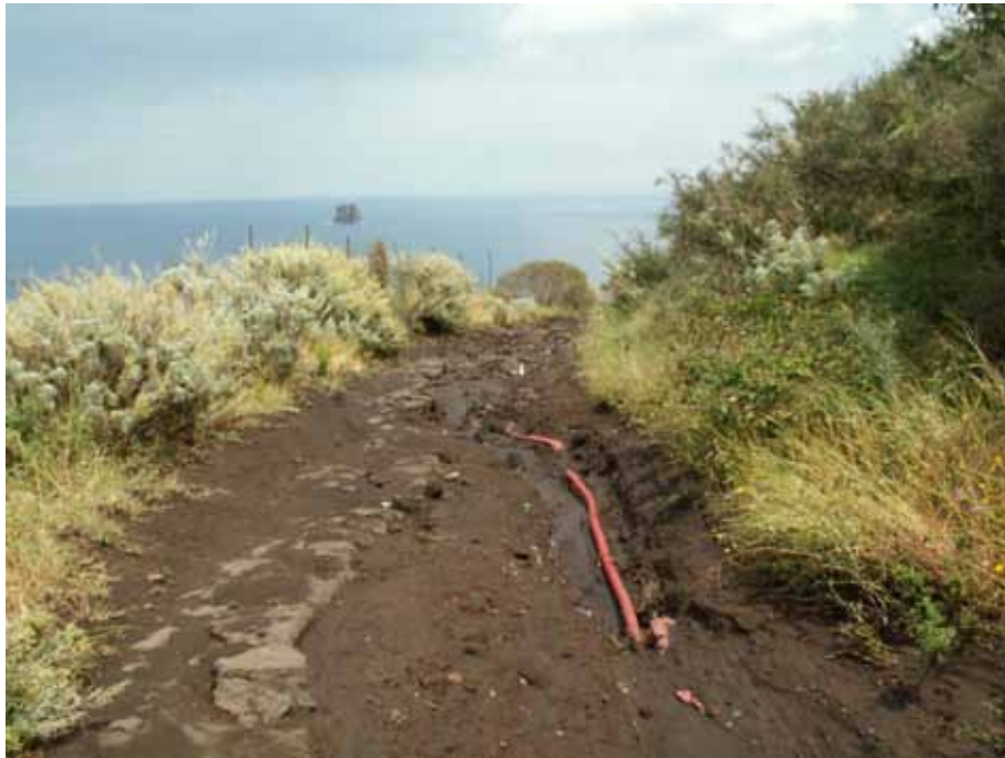
Figure 8.1: Buried-electrical and data transmission cables (May, 2007).
