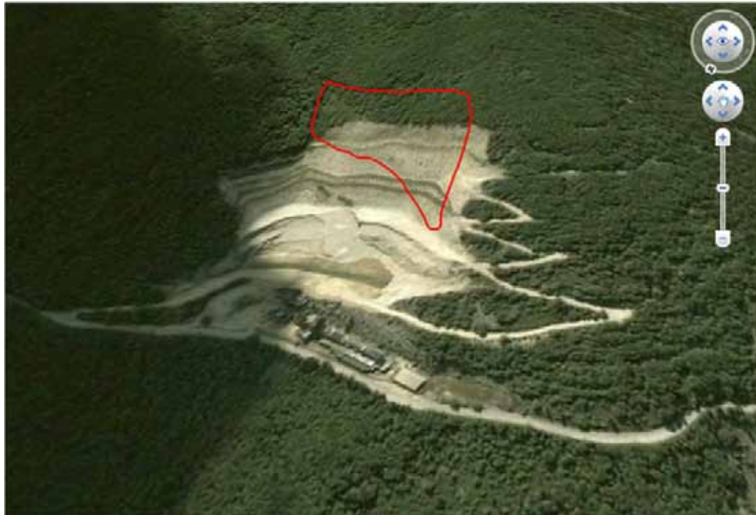
Figure 6.2: Photograph of the quarry and delimitation of the landslide (modified from [78]).
