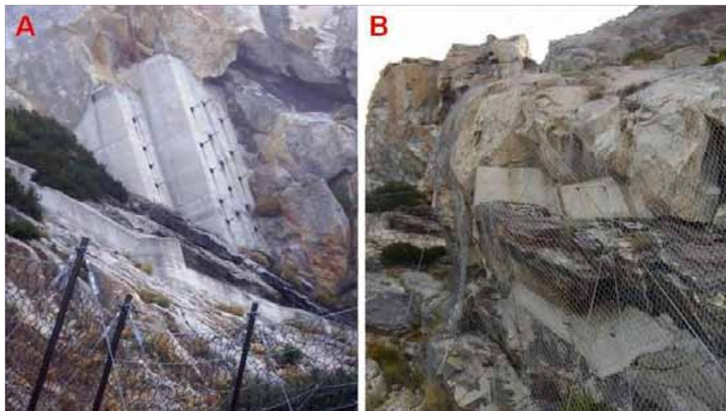
Figure 7.11: Underpinned structures (A) and beads (B) relating to the intervention of 88-'89 (April, 2010).
