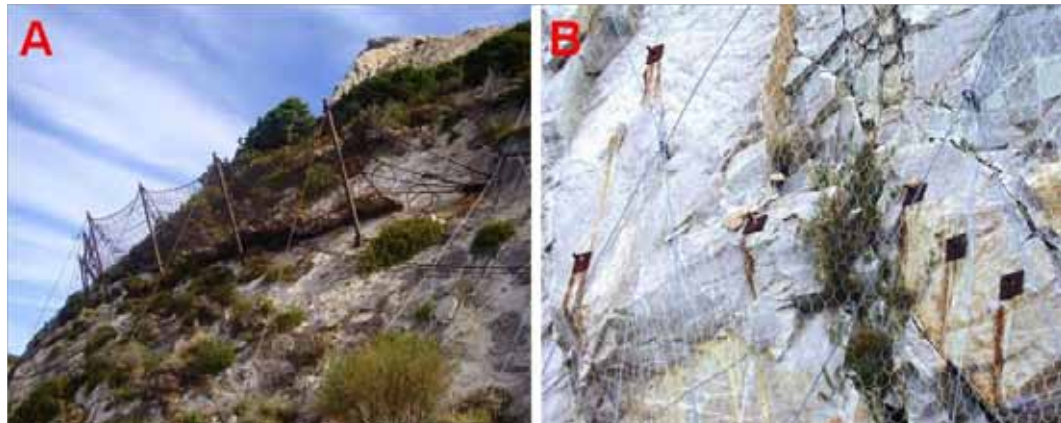
Figure 7.9: Rockfall protection installed in 1986 A-B); nailing surface.s '88-'89 (April, 2010).
