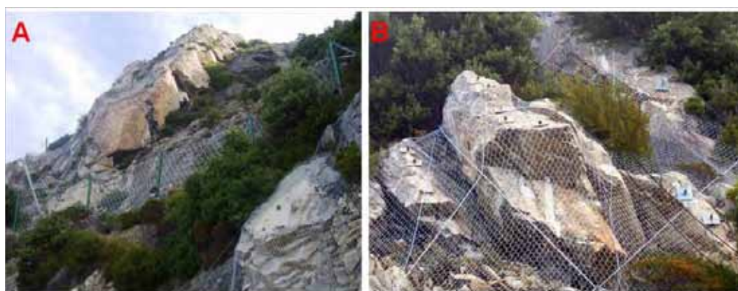
Figure 7.12: Rockfall protection installed in 1986 (A); nailing surface installed during the years (B) '97-'98 (April, 2010).
