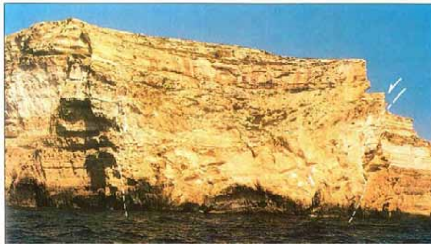
Figure 5.15: Collapse structure at the southern headland of San Dimitri Point, Gozo (taken from [66]).
