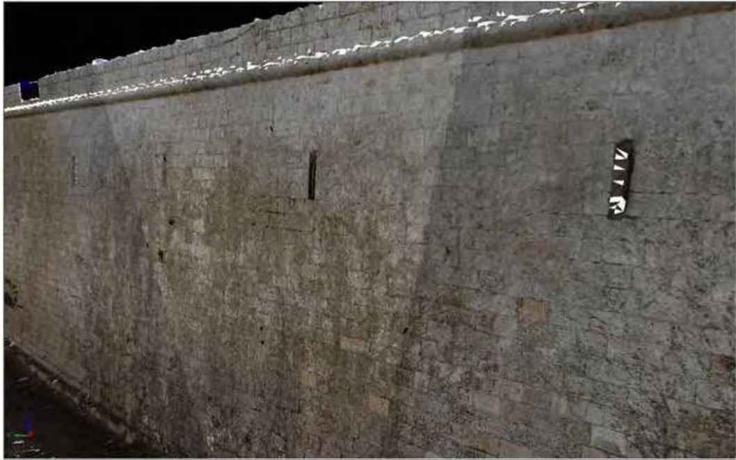
Figure 4.29: Area C. True coloured point cloud of the Magazine Curtain.
