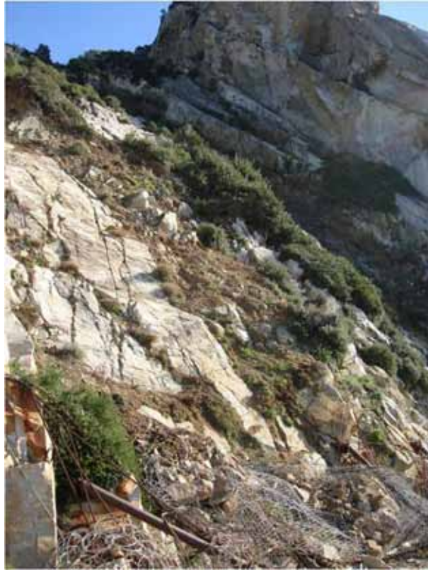
Figure 7.19: Debris flow along the impluvium separating rockmass 2 and rockmass event of 26 th December 2008 (May, 2010).
