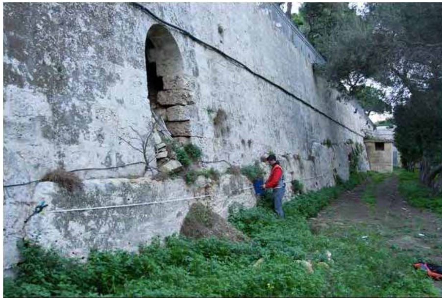
Figure 4.13: Geomechanical survey: Scanline 1 (December, 2007).
