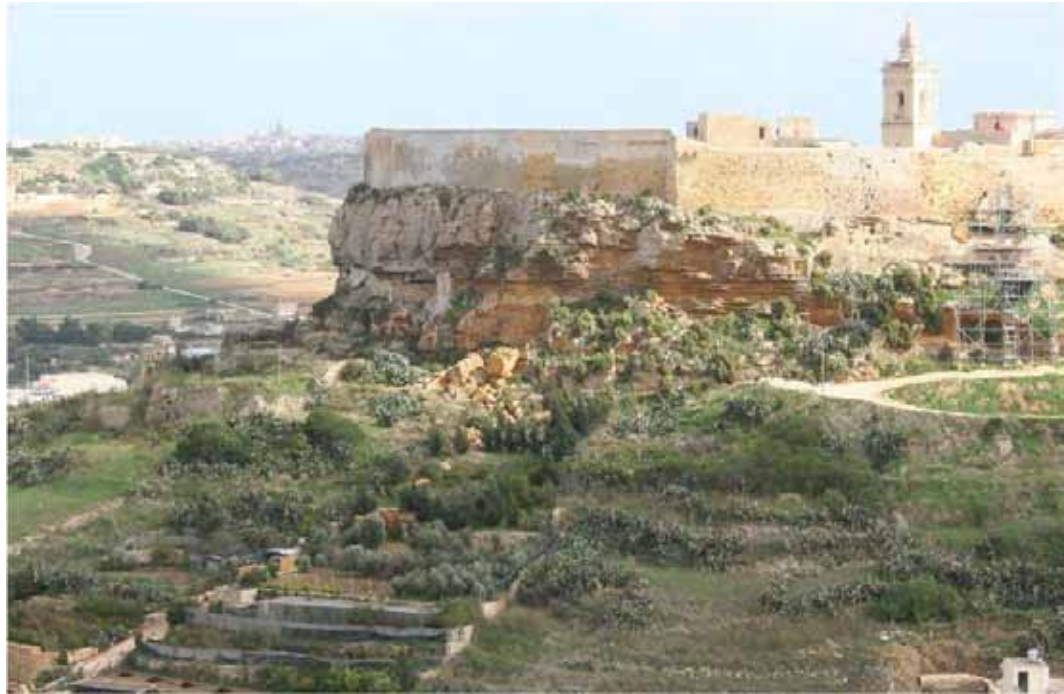
Figure 5.22: Rockfall debris from the 2001 event (May, 2010).
